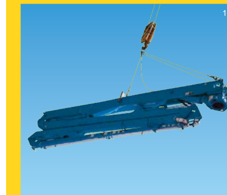
Step 3: Fly boom from truck to tower
