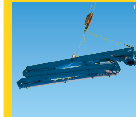
Step 3: Fly boom from truck to tower
